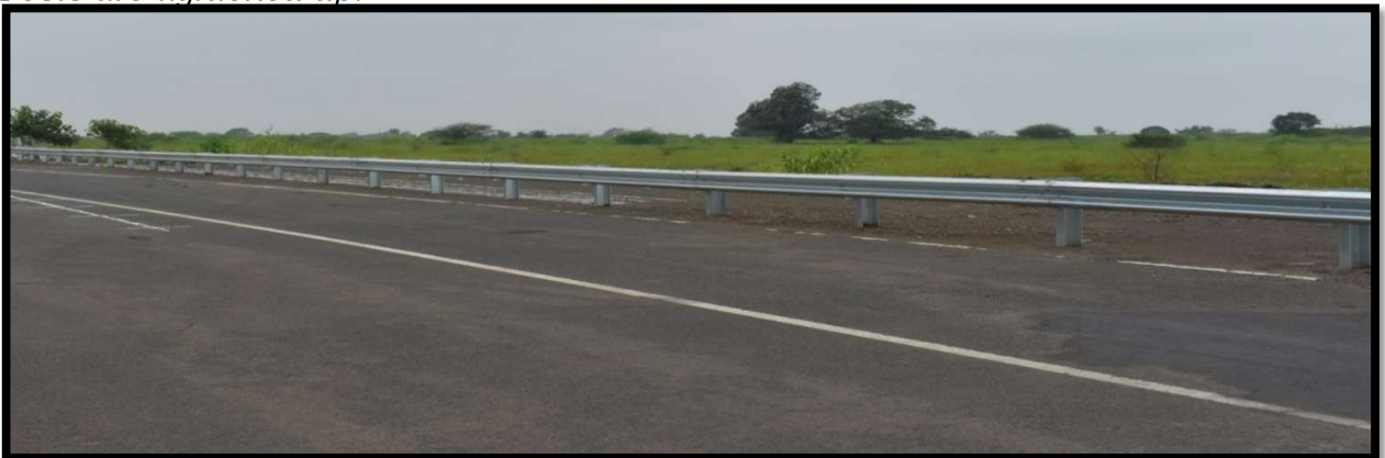
Over all View of Front side beam
