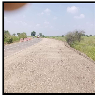
Area Compaction with 10 Ton Roller Compactor
