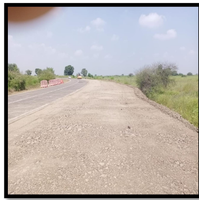
Area Compaction with 10 Ton Roller Compactor
