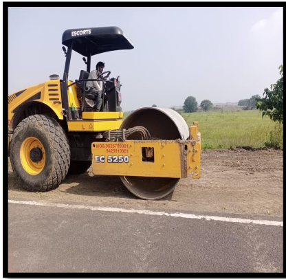
Area Compaction with 10 Ton Roller Compactor
