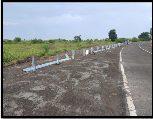
Insertion of remaining post and laying of beams in front of Barrier line
