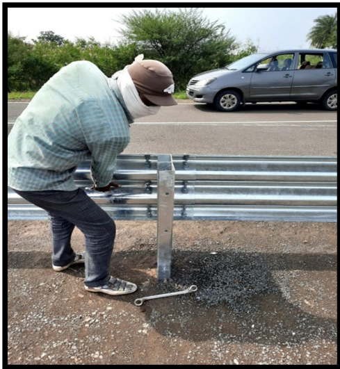
Insertion of remaining post and laying of beams in front of Barrier line
