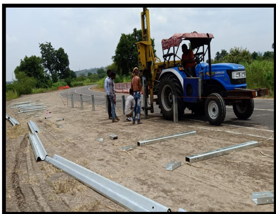
Insertion of end terminal posts as per depth required
