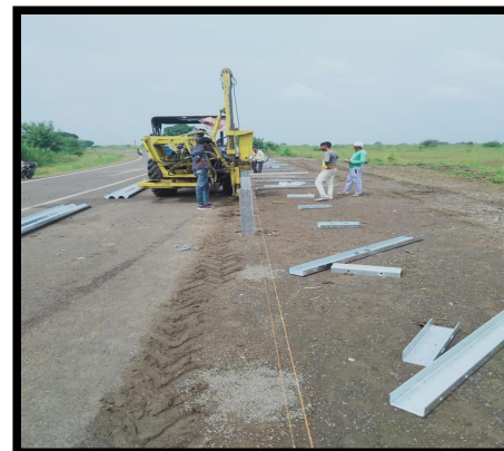
Insertion of end terminal posts as per depth required
