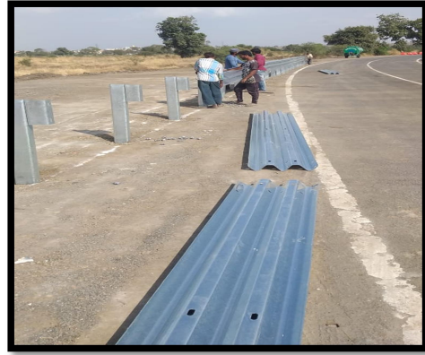
Insertion of remaining post and laying of beams in front of Barrier line
